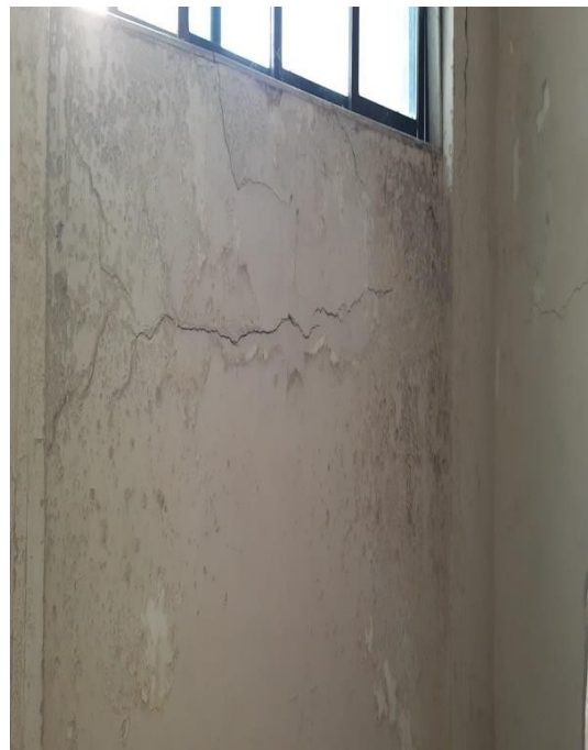
Corrosion crack has been observed on lintel beam.
