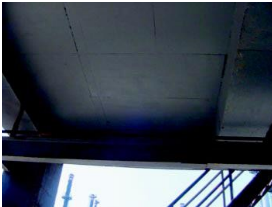
Fig: 17 Slab shuttering in position
