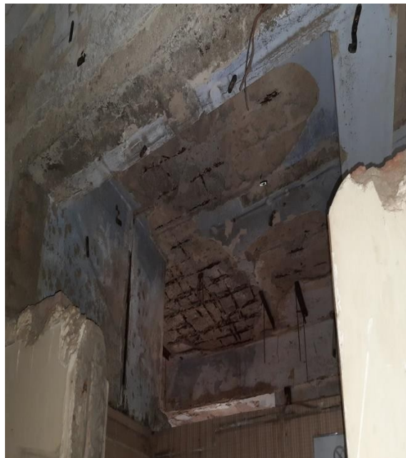
At most of the locations, spilling of cover concrete & exposed corroded & broken reinforcement has been observed on slab.
