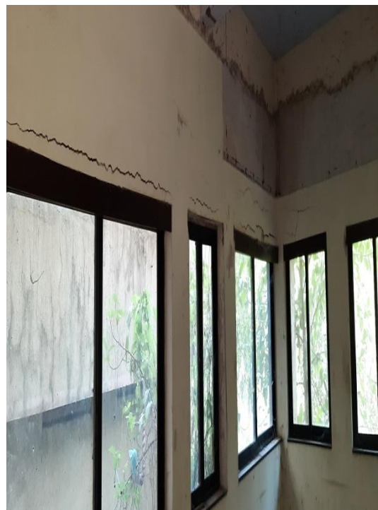
Wide corrosion crack has been observed at lintel beams.
