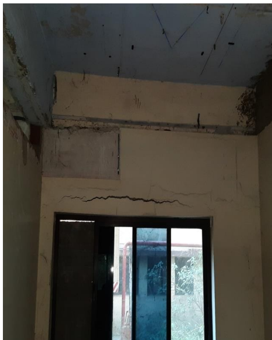
Wide corrosion crack has been observed at lintel beams.
