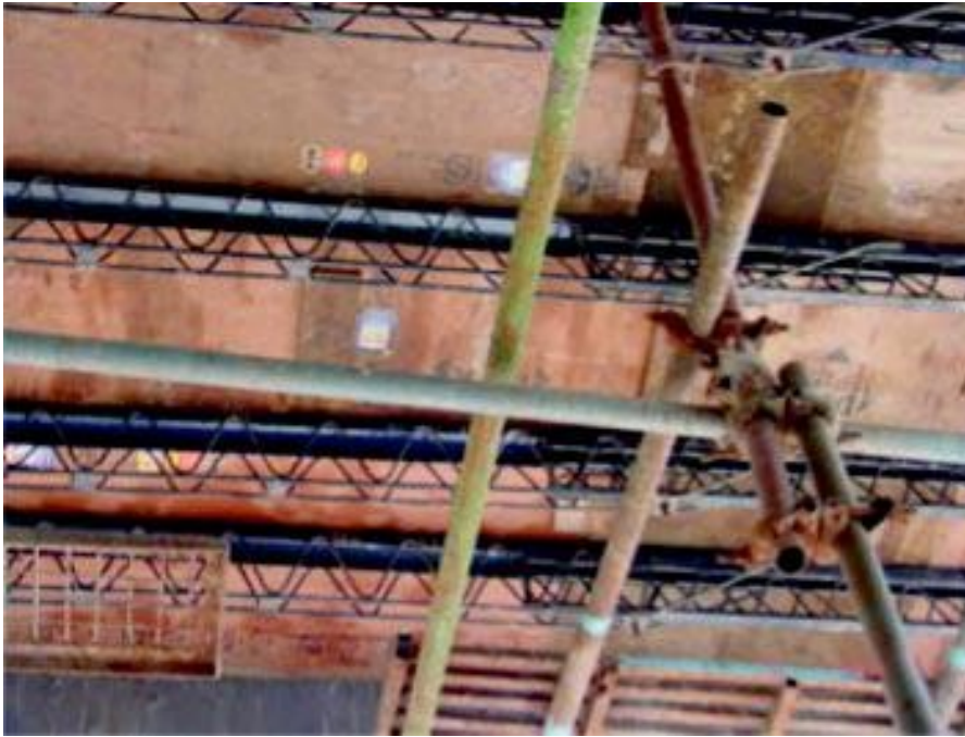
Fig: 17 Slab shuttering in position
