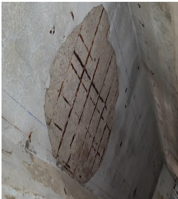
At most of the locations, spilling of cover concrete & exposed corroded & broken reinforcement has been observed on slab.
