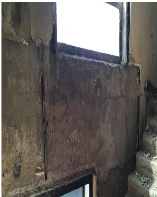
Corrosion crack has been observed on lintel beam.
